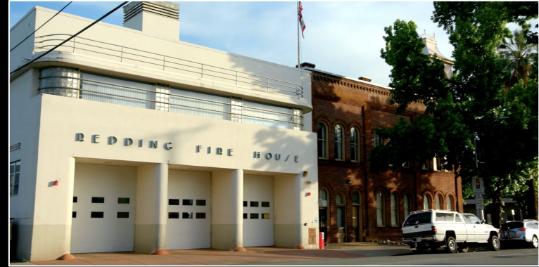
Siemens - City of Redding
